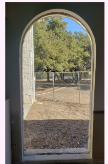
Window frame-out awaiting Stain Glass
